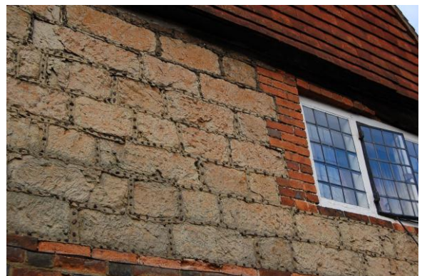
Figure 12: Photograph of the architectural technique 'galletting'
