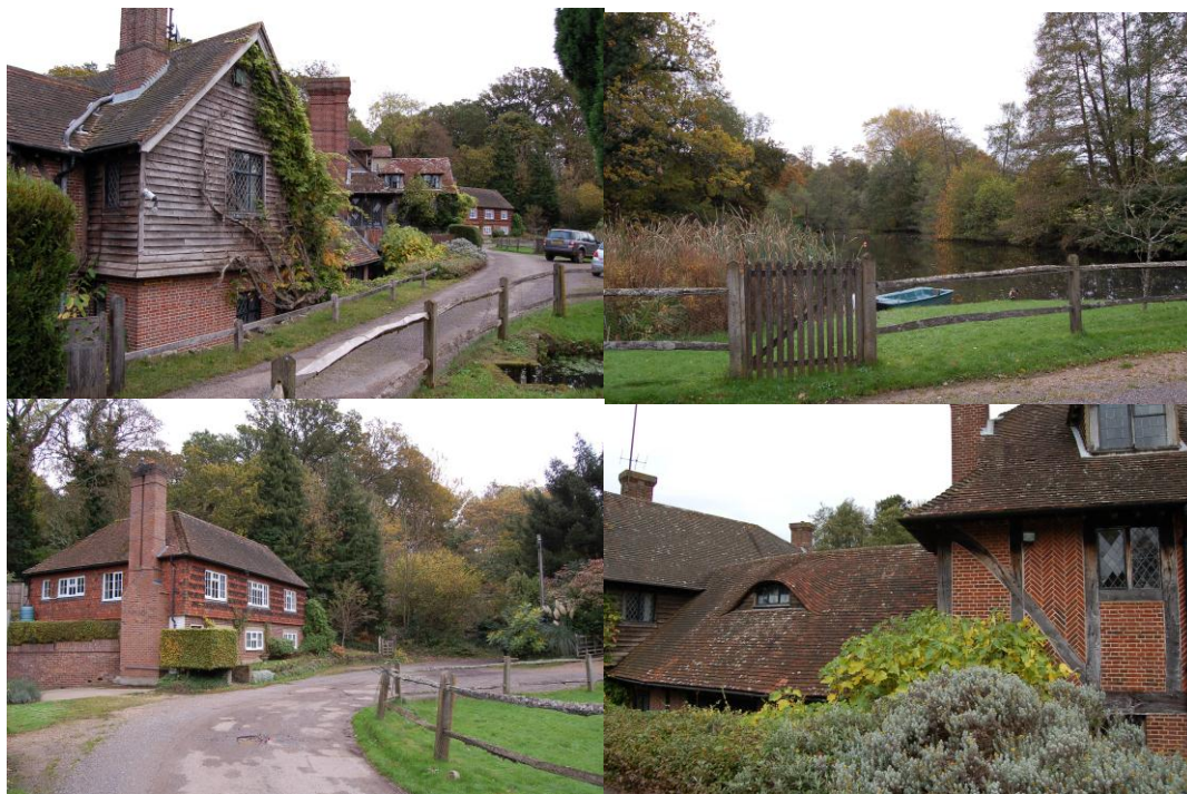
Figure 15: Top left: Enton Mill; Top right: Enton Mill ponds; Bottom left: Cobury Cottage and the disguised railway line behind; Bottom right: example of the architectural significance: eyebrow dormer, timber frames and brick nogging.
