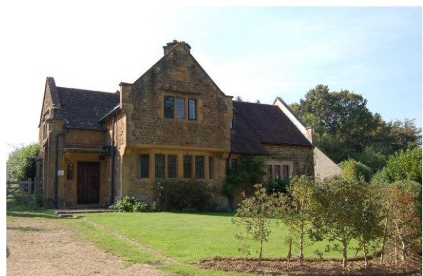
Figure 18: Witley Lodge, Churchfields
